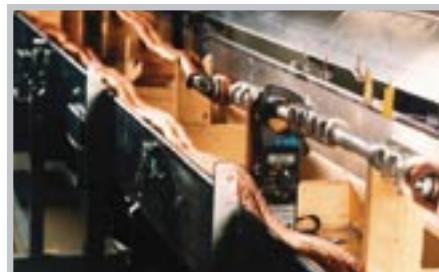
**Crimping is a System Technology. This means that it is the combination of a chosen terminal or connector and a matching crimp tool, all determined by the specific conductor that will result in the desired connection properties.**
